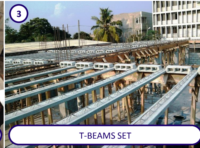
2 SETTING T-BEAMS ON THE STRUCTURE
